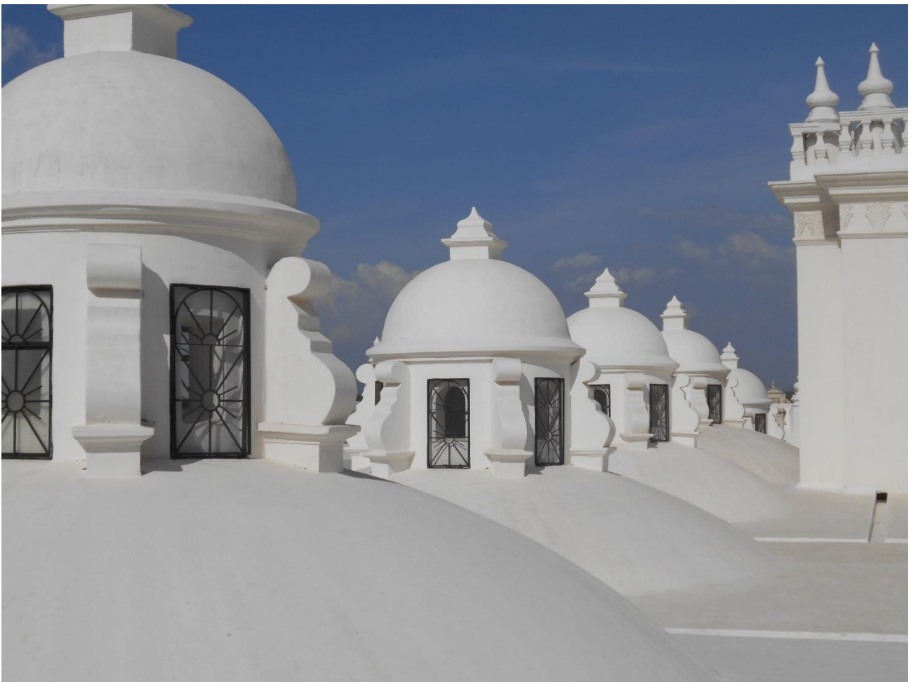
The cathedral roof – Leon, Nicaragua
